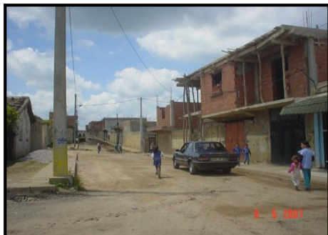
Route mal entretenue
