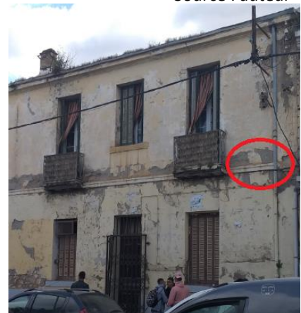
Figure 40.bandeaux simple
