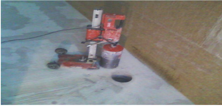
Figure I.11 La Carotteuse.
