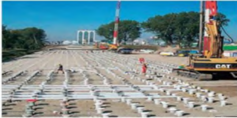
Figure 3.6. Principe Installation des drains.
