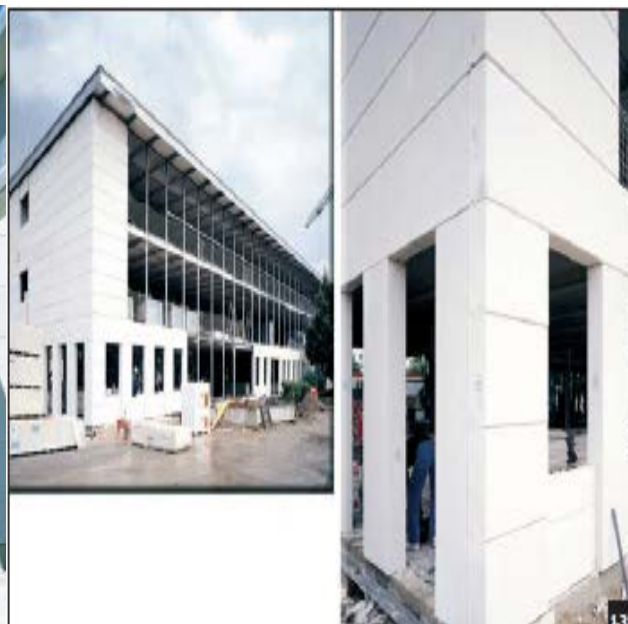
Figure III.5: Panneaux de façade [1]
