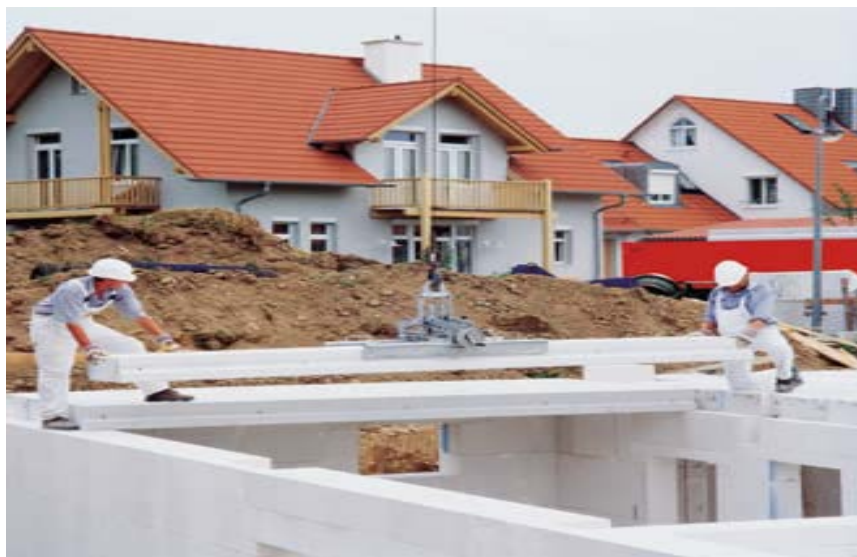
Figure III.7: Dalles de plancher [1]
