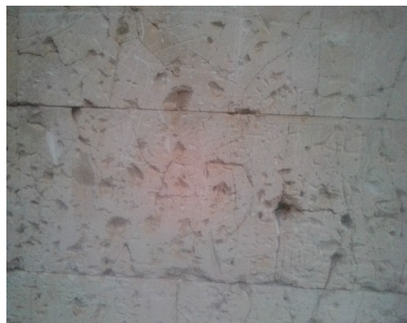
Figure V.6: Photo agrandie du mur
