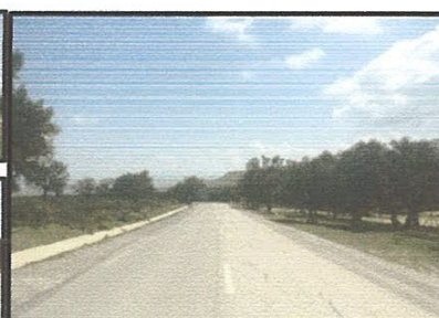
Figure 50: La route wilaya N 162
