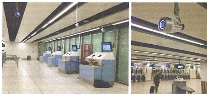
Figure 2.4: Passenger Flow and Queue Measurement : A Video surveillance system in London Gatwick Airport for counting passengers flow. (it counts near 10 million passengers per annum).
