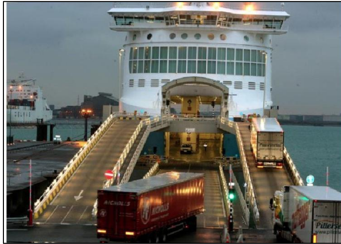
Figure 7 : Terminal routier, Dunkerque
