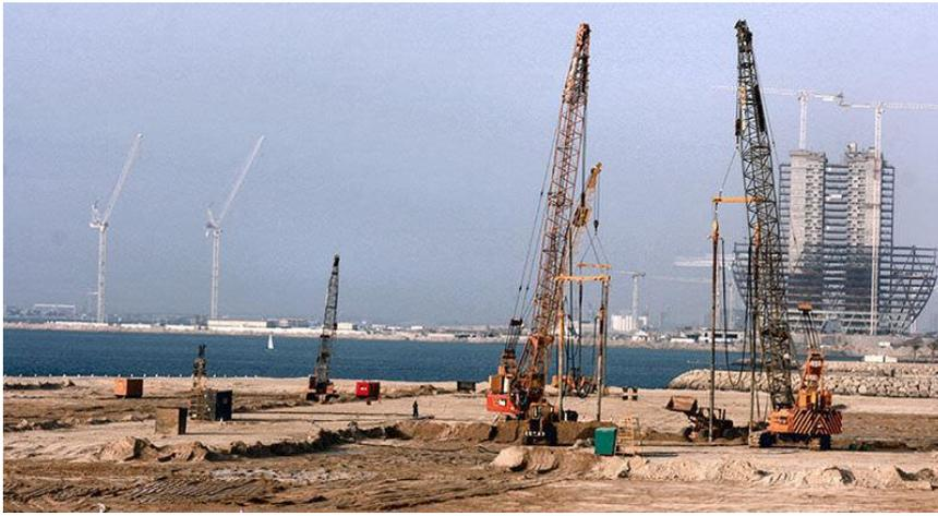
Figure 48: Vibrocompactage
