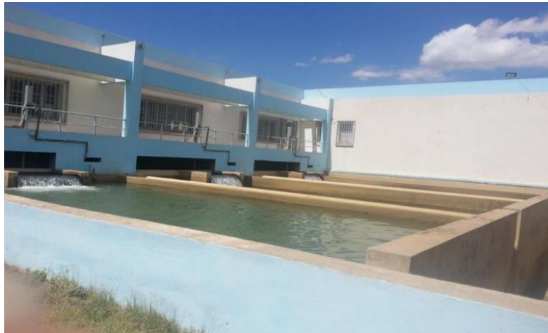
Figure II. 6. Bassin de filtration.
