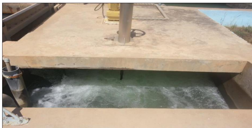
Figure II. 3. Bassin de coagulation
