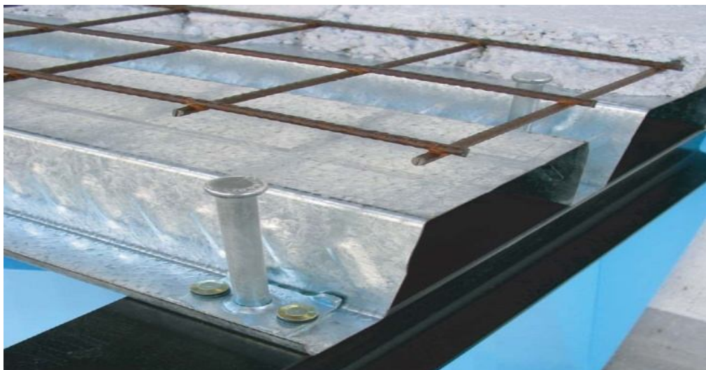
Figure VI.3: Treillis soudé
