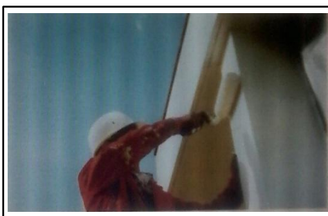
Photo III.4.6 : Application de la finition [66]
