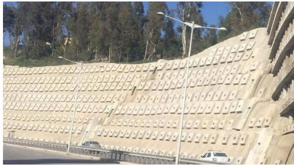
Figure III.5 - Un murs cloué : Mansora, Constantine
