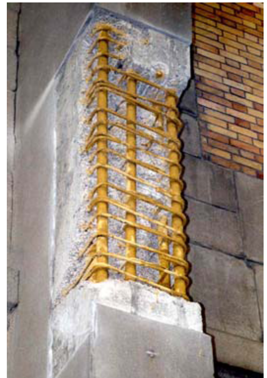
Fig I.28. Protection des armatures [J1]
