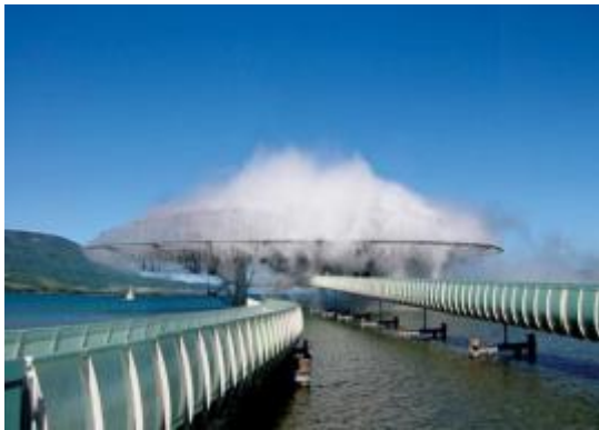
Fig 2.1 The blur building A lightweight metal structure sprays water and creates a unique atmosphere. Image source: http://www.dillerscofidio.com/blur.html
