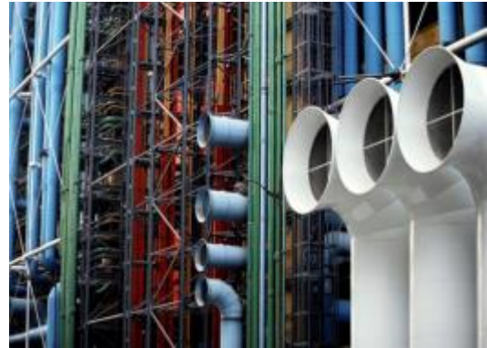
Fig 2.6 George pompidou center Renzo Piano, Richard Rogers In 2007 when reporting about the Roger's Pritzker prize the New York Times stated the design "turned the architecture world upside down".
