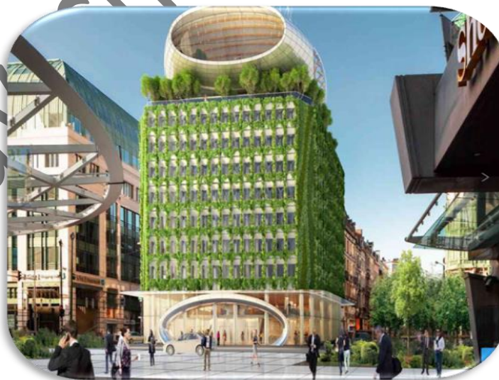
Fig 3.3 The Botanic Center Bloom Brussels, Belgium – 2016 (source: vincentcallebaut.com)
