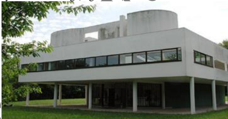
Fig 2.4 Villa Savoy by Le Corbusier Because the façade is free from structure, the windows can be continuous to create a panoramic view to the exterior landscape. It creates a visual continuity between the interior and exterior.
