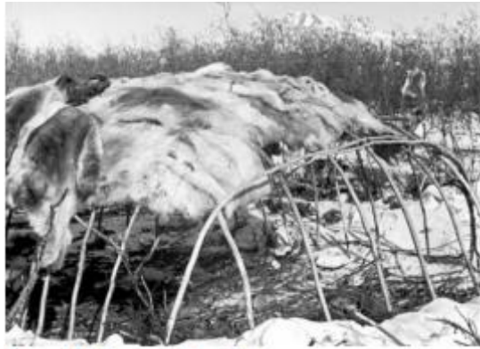
Fig 2.3 Caribou tent construction Photo Courtesy of Helge Ingstad
