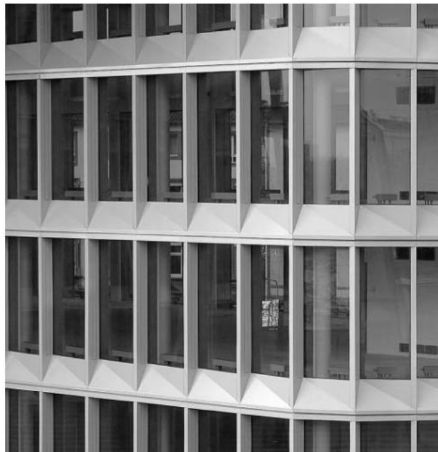
Figure 11: Westhafen Haus, Frankfurt, Schneider + Schumacher, 2005
