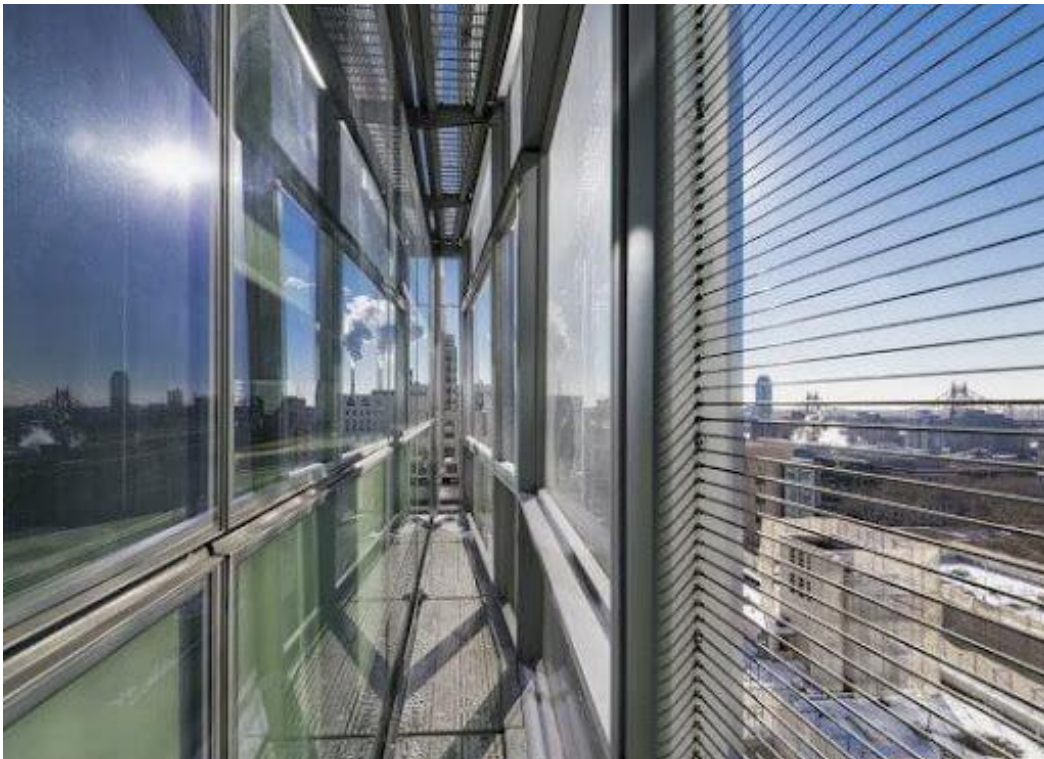
Figure 15: Detail of double skin façade.
