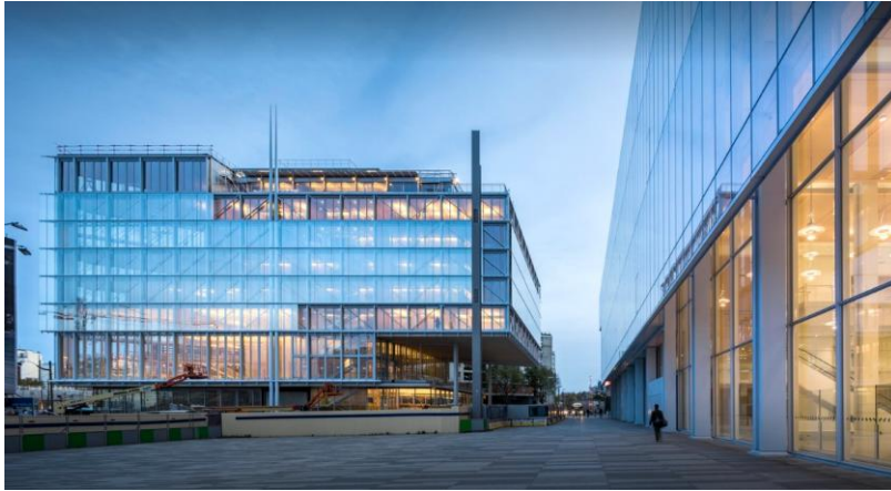
Figure 10: Curtain wall façade
