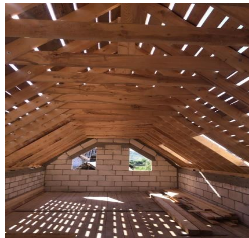
Figure 8: Charpente en bois [13]
