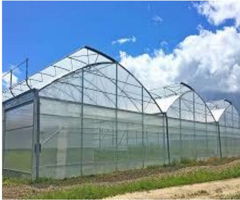
g). Double-Span ou multi-span
