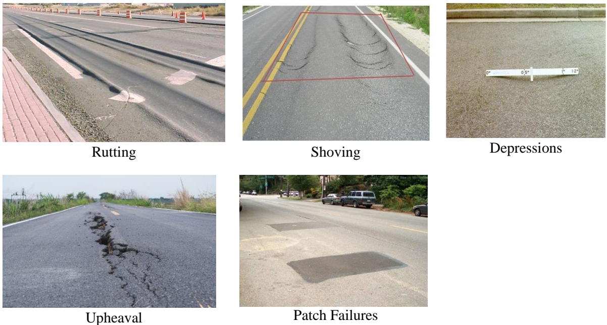
Figure 1.20. Types of distortion in asphalt pavement
