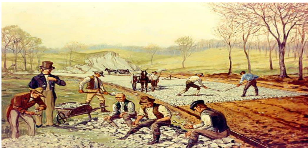
Figure 1.06. Construction of the first Macadamized Road in the United States (1823).
