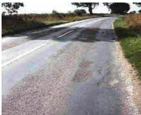
Loss of Cover Aggregate
