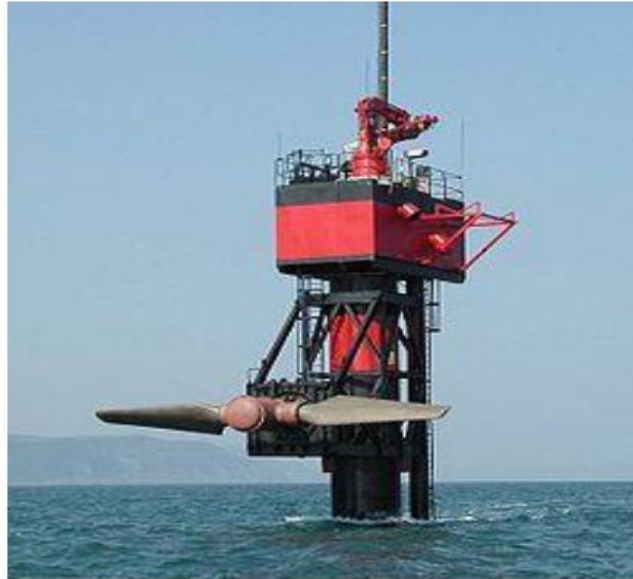
Figure (III.2): SeaFlow tidal turbine installed in north of Duvon, England [4].
