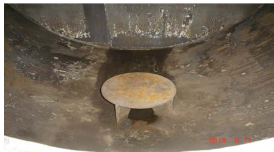
Figure II.12 : Anti-vortex [27].
