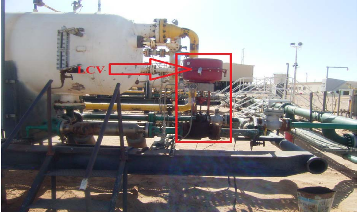
Figure III.7 : La vanne LCV.
