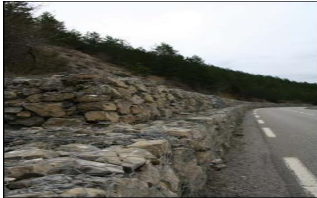
Figure .III.9 Structures semi-rigides
