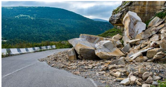
Figure. II.2 Chute de blocs. [12]
