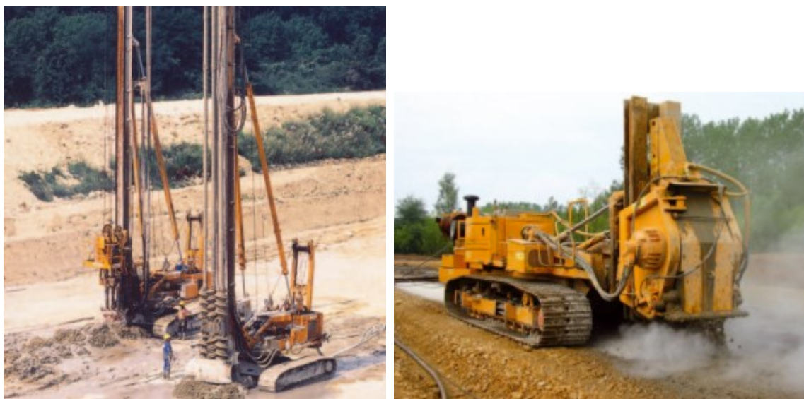
Figure I. 16. Outil de Jet Grouting.
