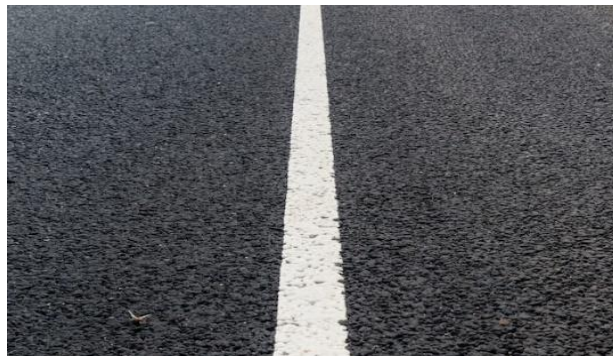
Figure IV- 11: Ligne Continue Blanche
