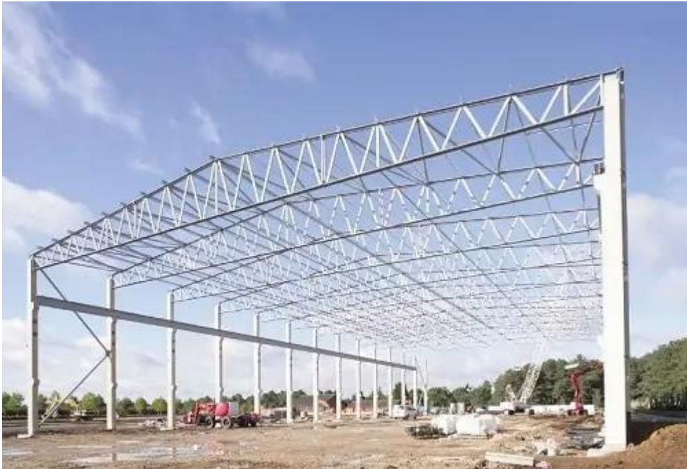
Figure 2: Structure en Acier.
