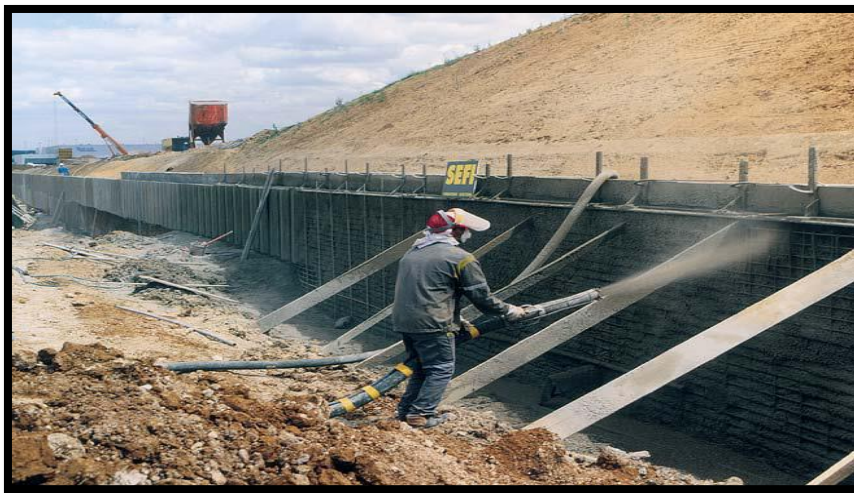
Figure I.13.Murs cloués
