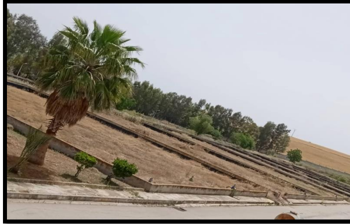
Figure II.10: Lits de séchage (STEP Guelma 2022).
