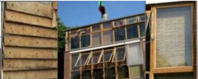
Figure 26: la protection solaire mobile
