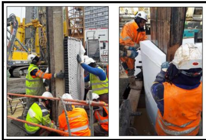
Figure II.21: Extraction d'une palplanche.
