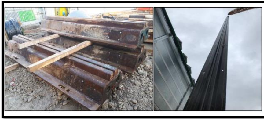
Figure II.20: Porte joint coffrage Water-Stop.
