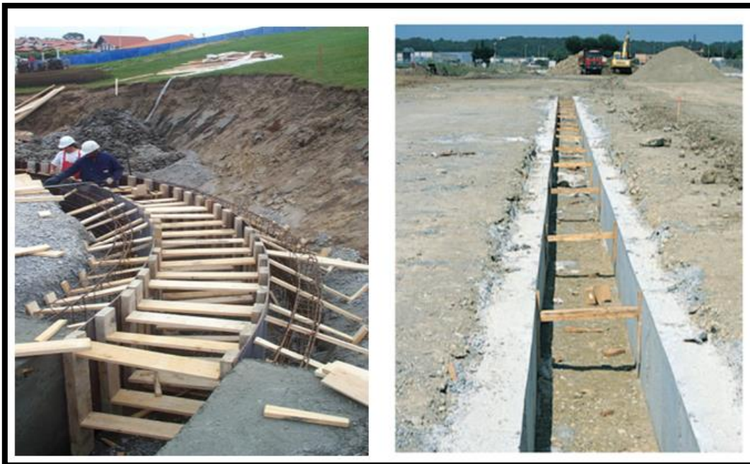
Figure II.5 : murets-guides circulaires.
