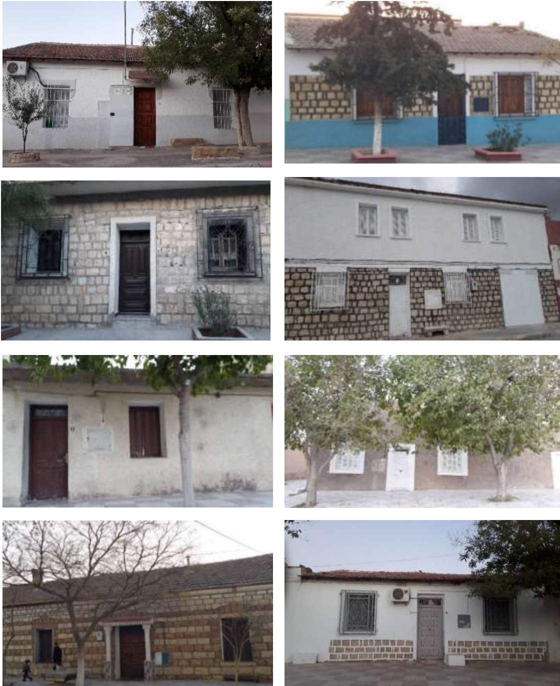
Fig. III.6. Ancient residential buildings in Tébessa ( Source: The Author )
