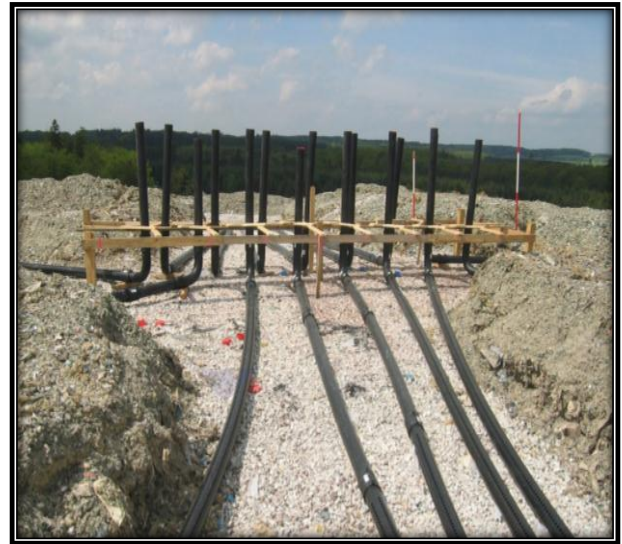
Figure 8 : Collecte du biogaz (drains horizontaux) (GIZ ,2016)
