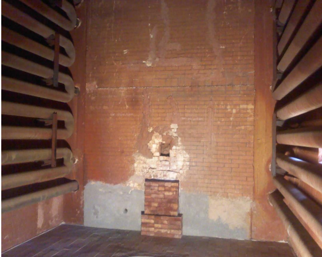
Figure II.3 : Serpentins du four topping.
