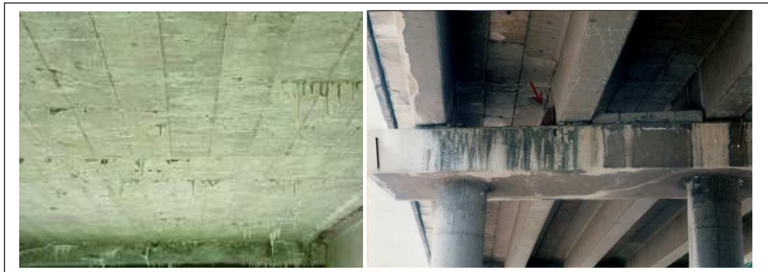
Figure I-29 : Efflorescence
