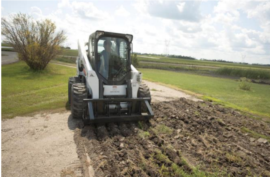
Figure 53: Scarification des sols
