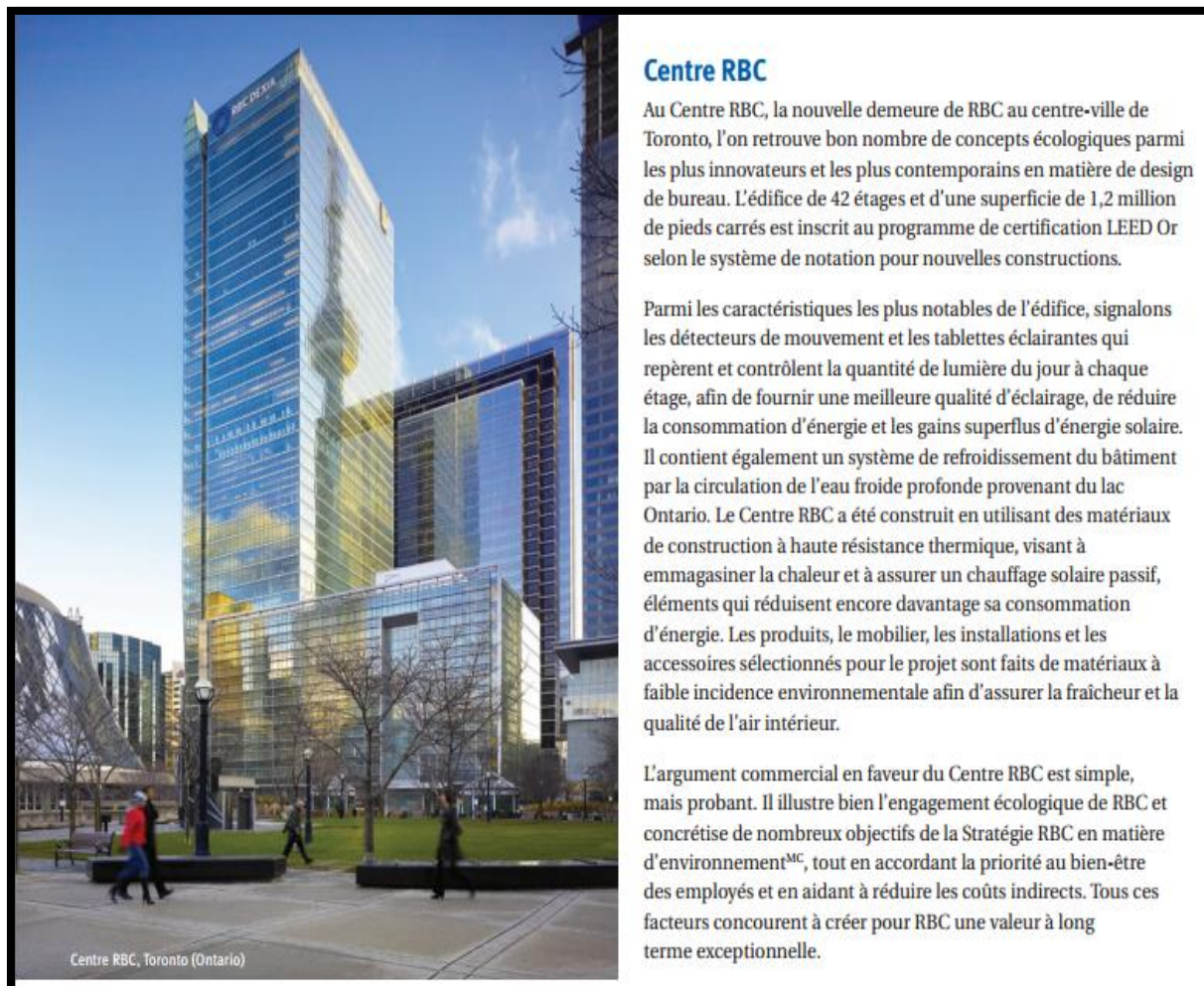
Figure 114: exemple de centre RBC
