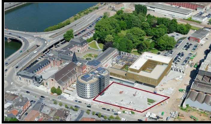
Figure 10: L'esplanade Kuborn –chantier
