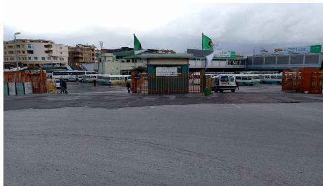
Figure 54: La gare de Jijel.
