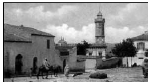
Figure 7 Mosqué EL ATIK https://addislighting.com
