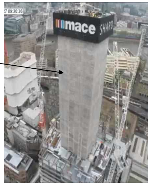
Figure 8 Le noyau en béton 04. Construction of The Shard (London Bridge Tower)
