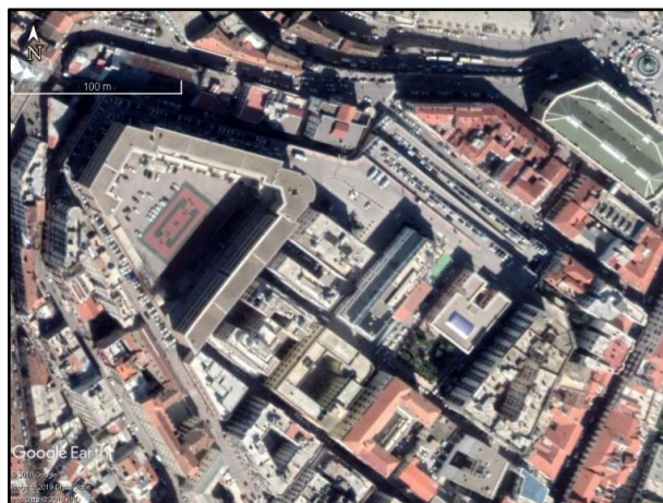
Figure IV- 13. Housing moderate rents in district of Coudia at the city of Constantine.
