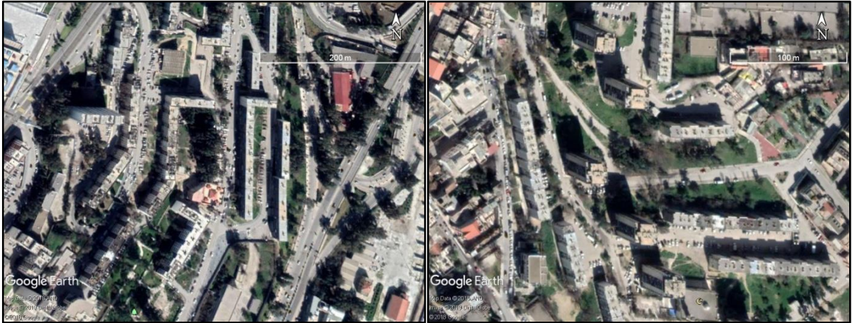
Figure IV- 16. Resettlement buildings of Fadilla Saadane houses in Belle Vue district (left) and Bousquet houses in Sidi Mabrouk (right) in the city of Constantine.
