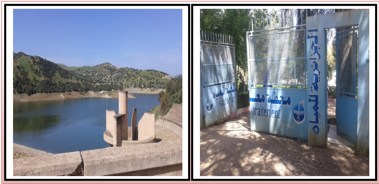
Figure 15: SP1 barrage Hammam Debeh (Source: NAILI .A & MENIDJEL .Y 2018)
