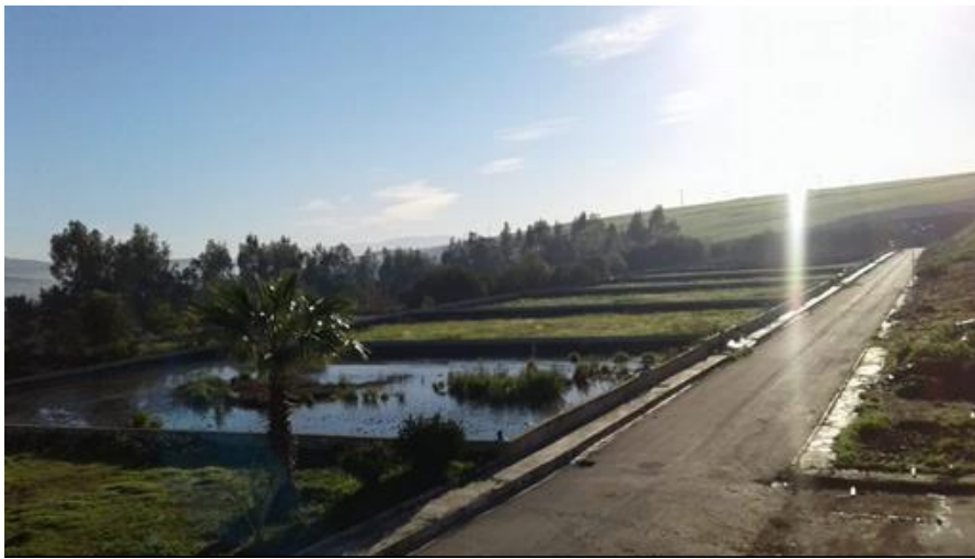
Figure II.10: Lit de séchage
