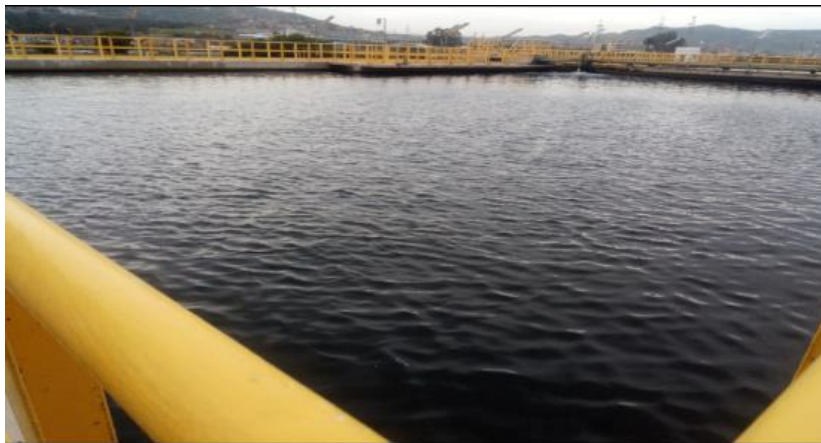
Figure II.11 : bassin de protection GP-1A/B
