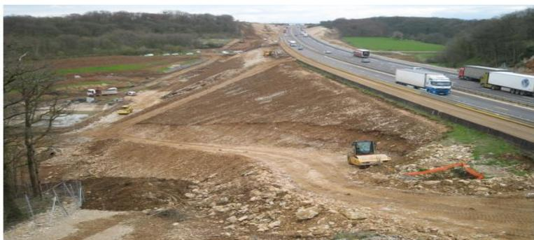
Figure II.2 Remblai routier [1]
