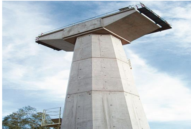
Figure .I.6 : Pont TGV Perpignan-Figueras. [1]
