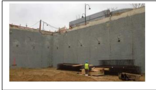
Figure II.24. Paroi moulée
