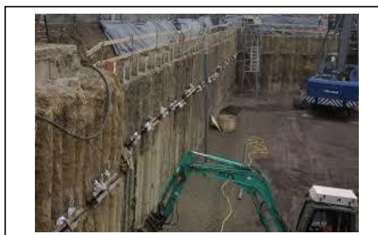
Figure II.25. Paroi du type mixed in place.
