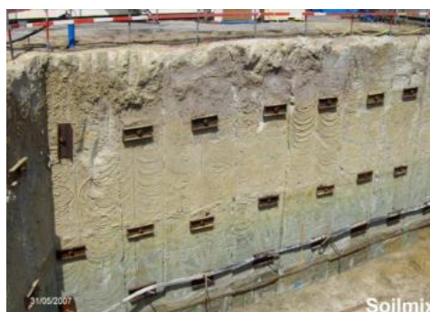
Figure II.26. Paroi du type cutter soil mix.
