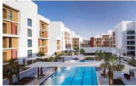
Figure 84 : Etihad Eco residence Source : https://www.archdaily.com/
