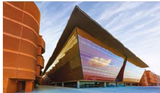
Figure 86: Incubator Building Source: https://www.archdaily.com/
