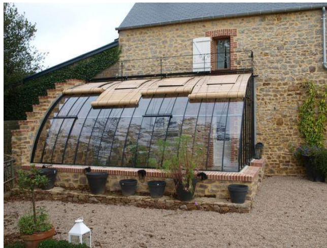
Figure 20: serre accolée, source : www.pinterest.jp
