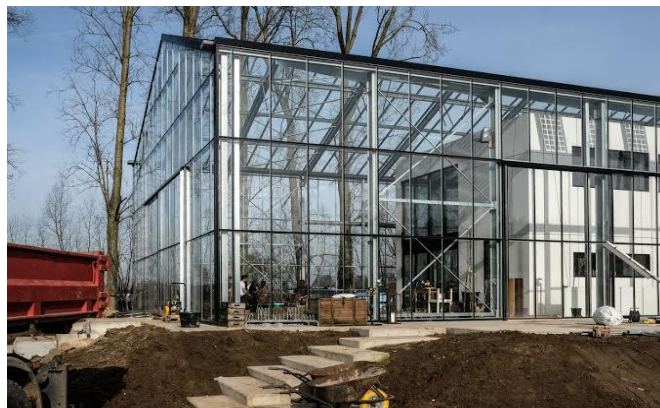
Figure 22: serre enveloppe source : www.build-green.fr
