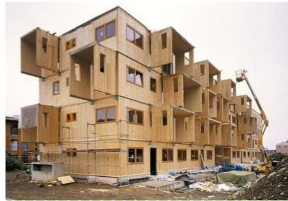
Figure II. 6: Structure en panneaux bois massive. Source : [26]
