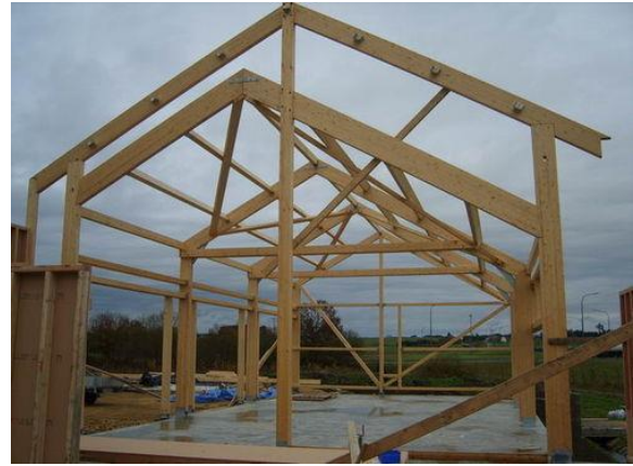
Figure II. 5: Maison poteaux-poutres. Source : [25]
