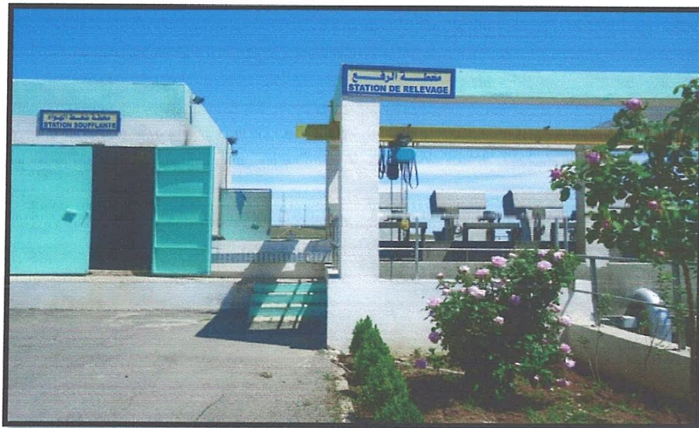
Photo I.1 : La station de relevage
