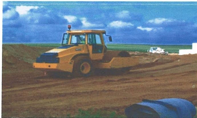
Photo4.1. operation de compactage
