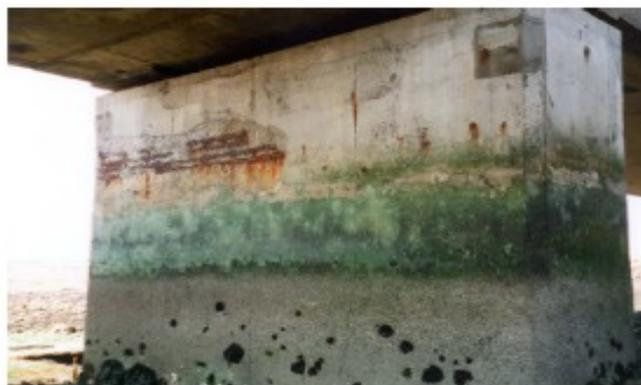
Figure I.1 : Erosion abrasion cavitation [AFG-11].
